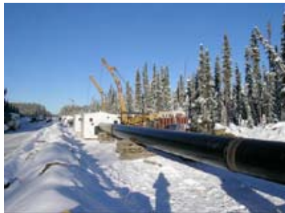
Pipeline Construction in L 690 (X100) High Strength Line Pipe (Canada)
